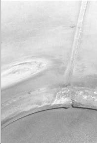
Overheating, stress crack
